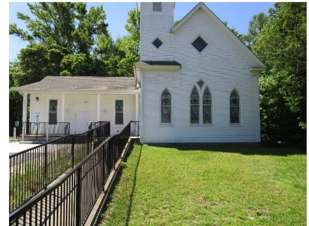
A rain garden can be installed in this area by connecting the downspout on the western side of the building to the location. A section of parking spaces can be converted to pervious pavement to capture and infiltrate stormwater runoff from the roof and parking lot. A preliminary soil assessment suggests that more soil testing would be required before determining the soil's suitability for green infrastructure.
