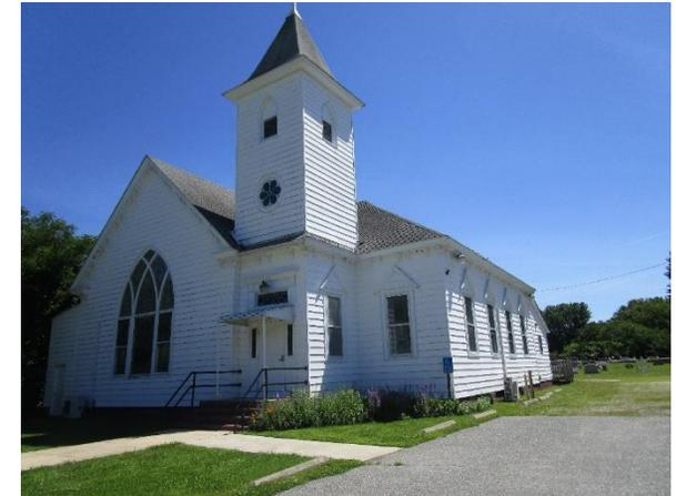
A rain garden can be installed in the front of the building. A connected downspout can be disconnected and redirected into the rain garden. A preliminary soil assessment suggests that more soil testing would be required before determining the soil's suitability for green infrastructure.
