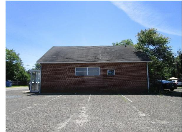
Pervious pavement can be installed in the parking lot to collect stormwater from the three downspouts from the eastern side of the building. A preliminary soil assessment suggests that more soil testing would be required before determining the soil's suitability for green infrastructure.
